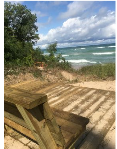
Ridge Beach Viewing Deck.
