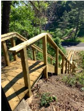
Crest Drive Stairs.
