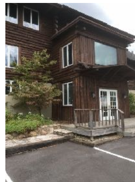
Clubhouse Exterior Refurb.
