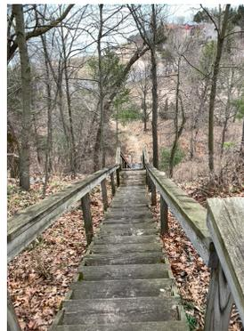
Two sets of aging (and not too safe!) beach access stairways are slated for removal . . . and replacement this summer! Both sets of stairs are at least 35 years old and the years and weather have taken their toll. Treads and railings have been replaced over the years, but for the sake of safety, the time has come for a complete reconstruction, including
